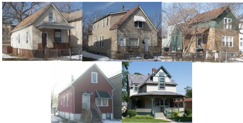
Figure 1. Frame homes included in project
